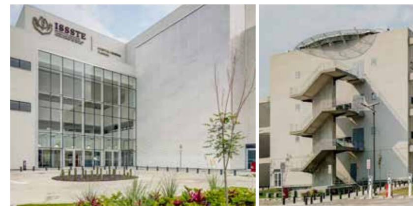
The Hospital de Tláhuac shortly before commissioning. Clearly discernible are the three buildings sharing one platform. The seismic isolators are installed underneath the platform.
